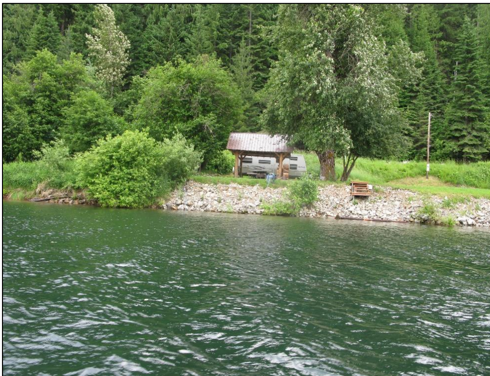
Figure 16. Completed construction, post-restoration June 2019.
