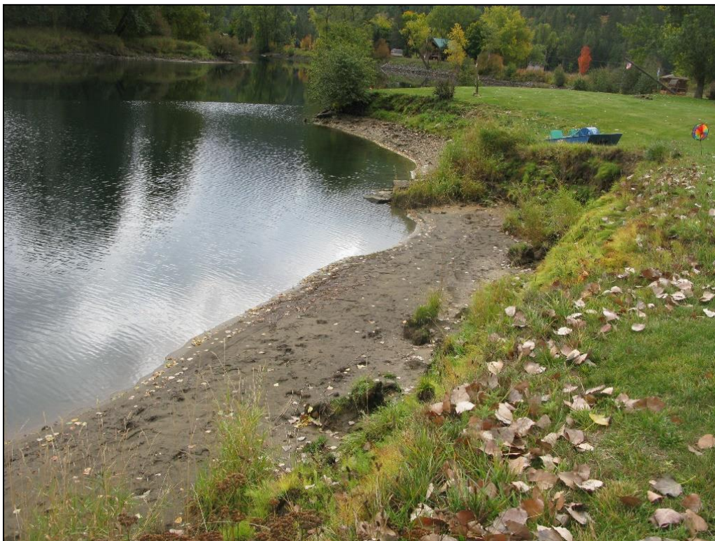
Figure 8. Tall, steep eroding banks and lack of riparian vegetation, pre-restoration October 2017.
