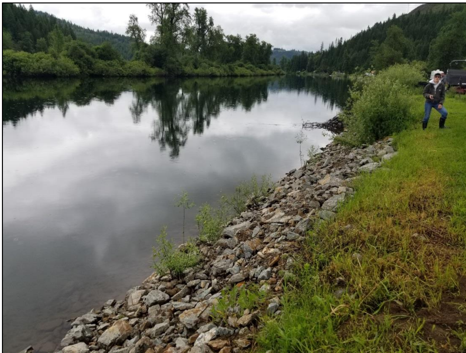
Figure 20. One of this project's newly planted sites in the foreground with a past NRCS project on the adjoining property upstream in the background, post-restoration June 2020.
