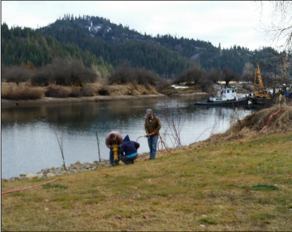
Figure 15. Planting willows with pneumatic driver, during construction December 2018.
