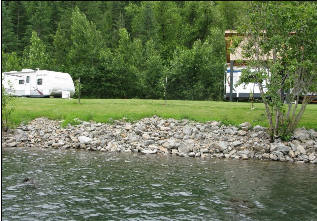
Figure 17. Willow bundles, rock, and cottonwoods, post-restoration June 2019.
