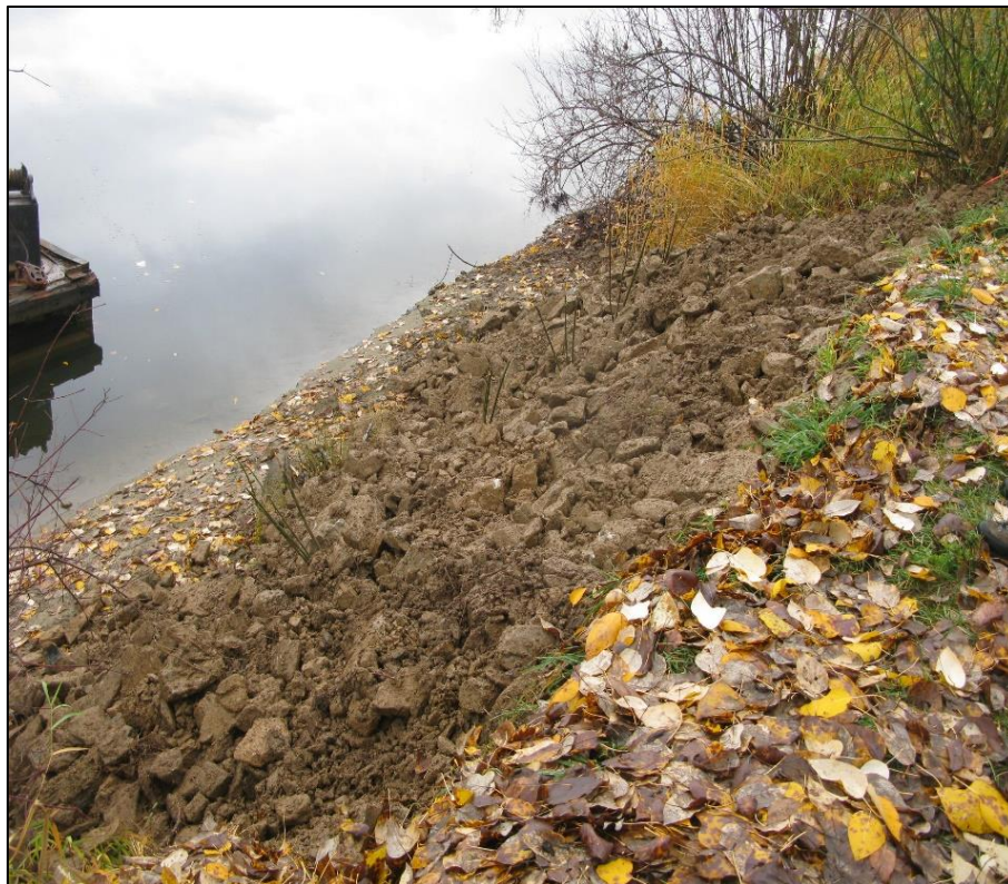
Figure 14. Willow bundles being planted with rock, during construction November 2018.
