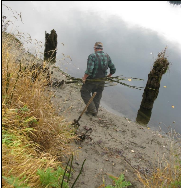
Figure 13. Willow planting, during construction November 2018.
