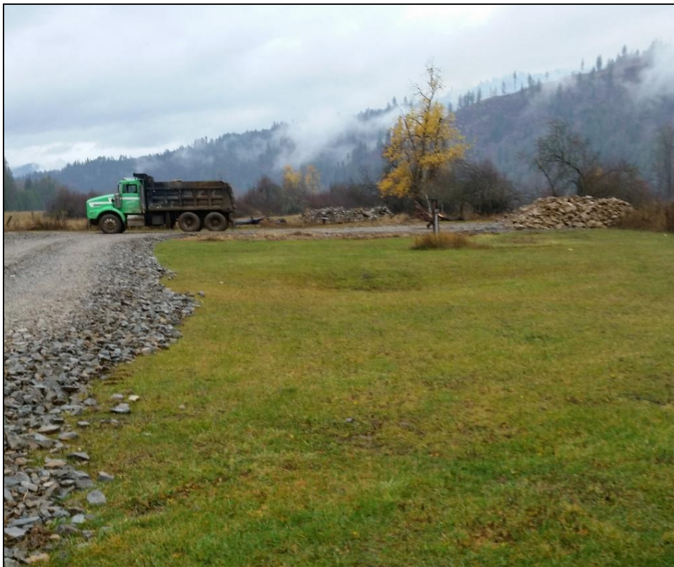
Figure 10. Access road and rock staging, during construction November 2018.
