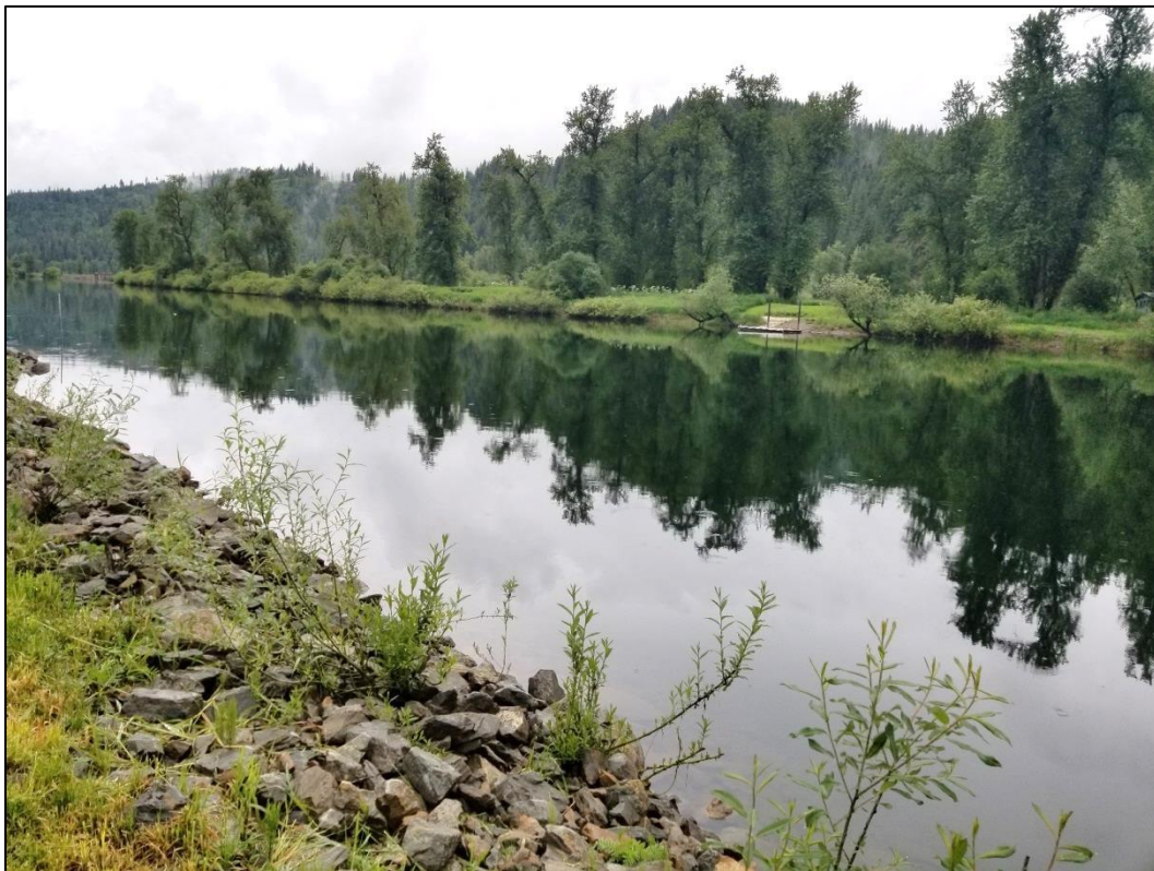
Figure 18. Willow bundles and rock, post-restoration June 2020.
