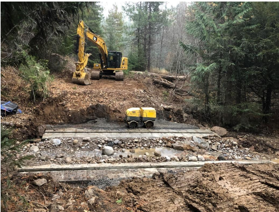
Photo 2. A simulated streambed was constructed between the two concrete footings. The slotted channel in the concrete footings on either side of the streambed that will hold the new culvert in place is clearly visible in this photo.
