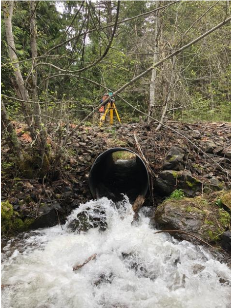
Photo 1. The former upper Lake Creek stream crossing that was identified as a fish barrier.
