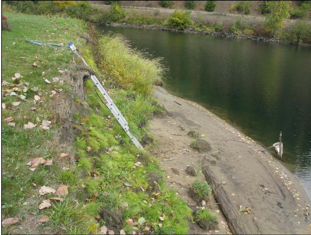
Figure 7. Tall, steep eroding banks and lack of riparian vegetation, pre-restoration October 2017.
