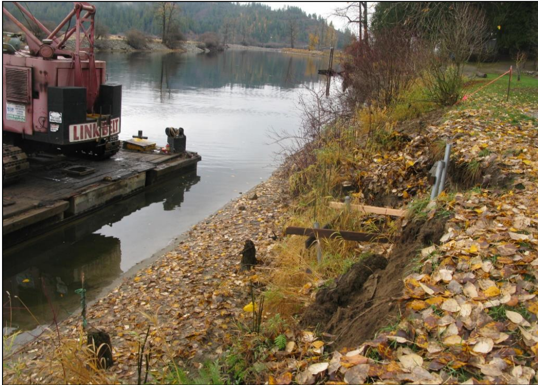
Figure 12. Beginning construction, during construction November 2018.
