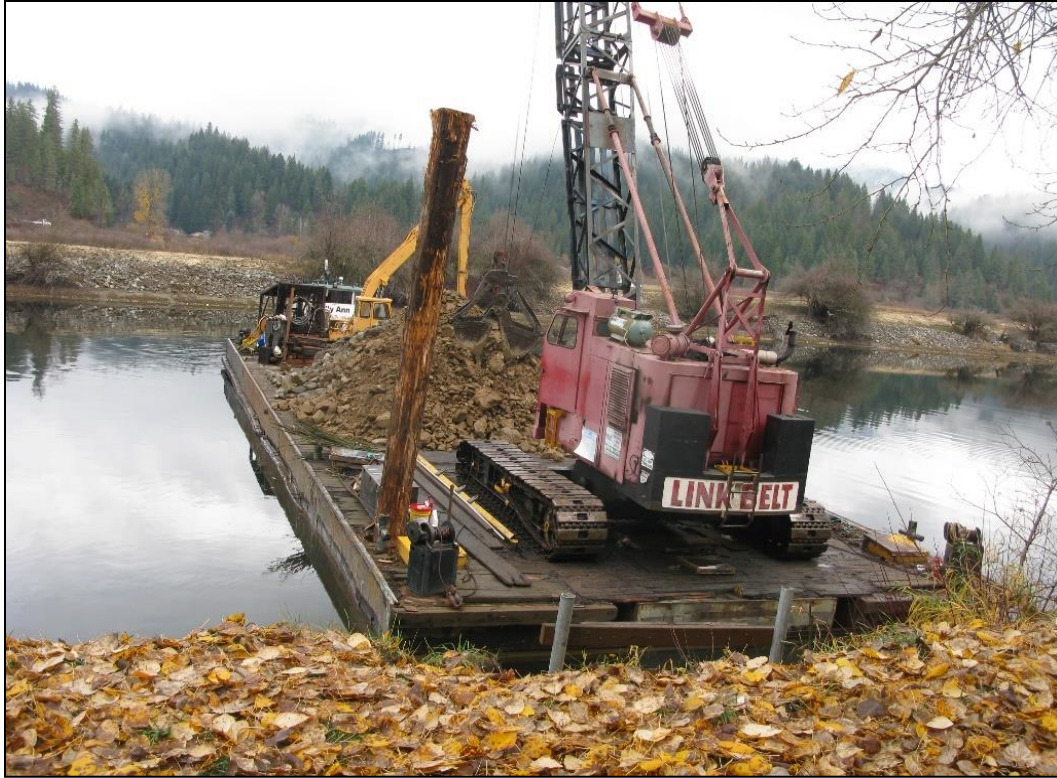
Figure 11. Barge for construction, during construction November 2018.
