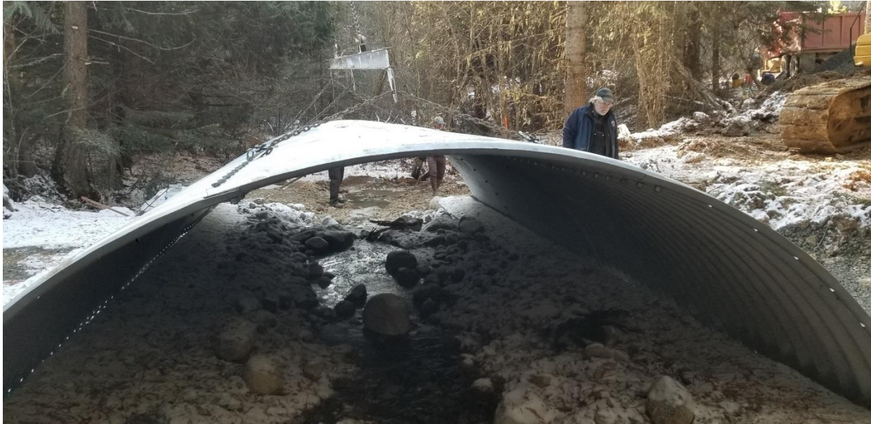
Photo 3. The plate arch culvert was pieced together then lifted on to the concrete footers to finish the job of constructing the new passage structure.
